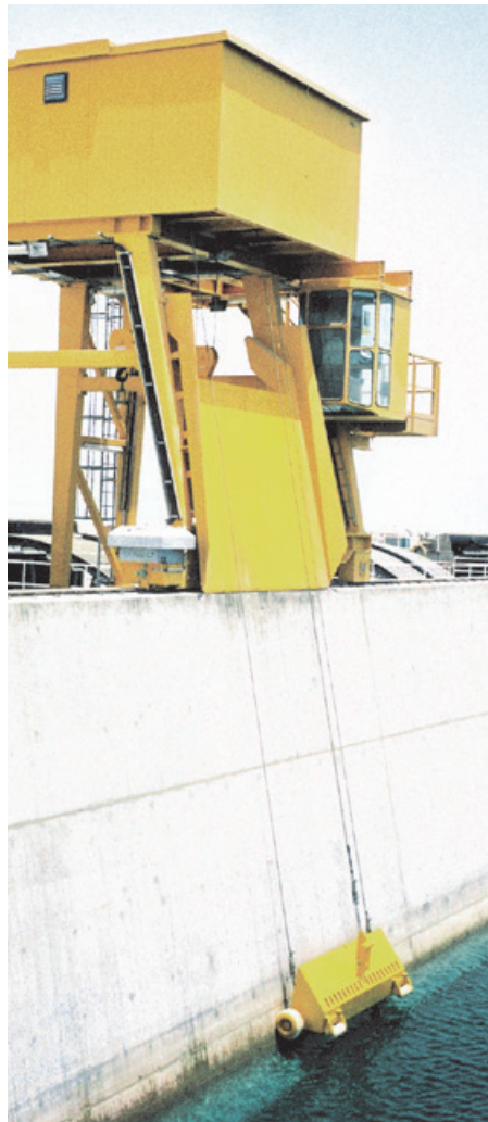
Picture bottom right: Passavant®/Geiger® Traversing Cable- Operated Grab Cleaner in Action at a Plant in Sweden
