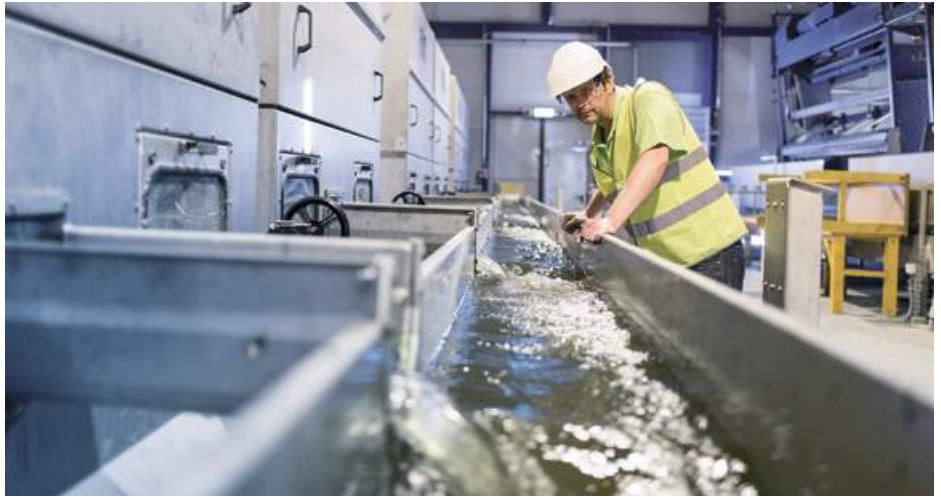
Power Plant Intake in Europe: Geiger MultiDisc® with Fish Trough and Cover Panels
