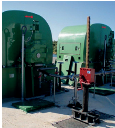
Travelling Band Screen Dual Flow Pattern
